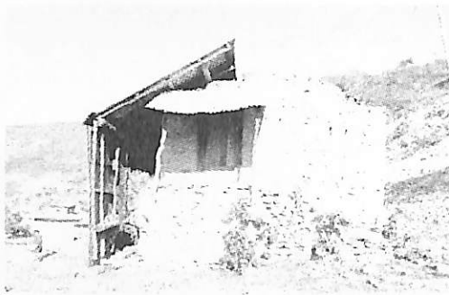
Fig.4 Wind damaged roofs(2011)
